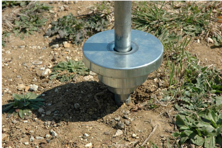
Figure 5.6 Penetration of DCP Equipment into the Pavement Courses
