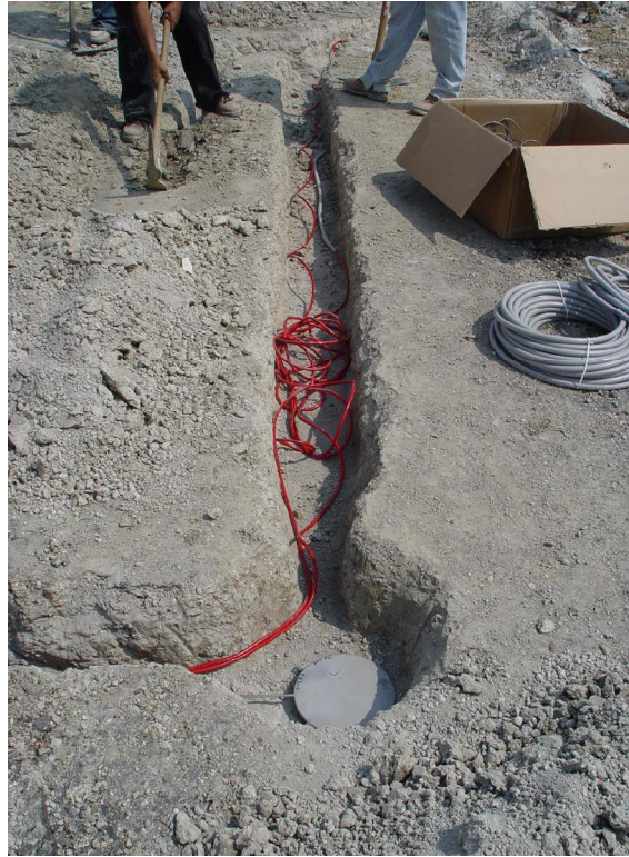
Figure 4.5 Placement of Pressure Cells (Pillappa, 2005)
