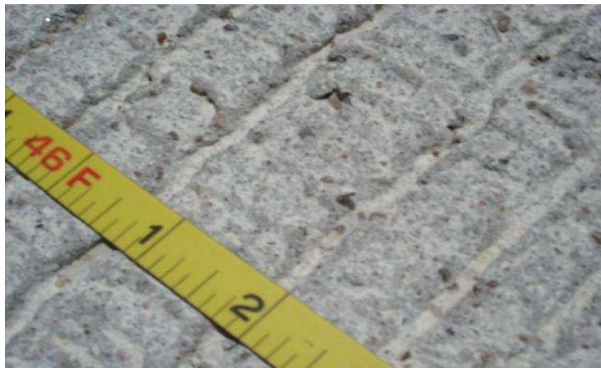
Figure 5.38 Tinning from section measured from SH130
