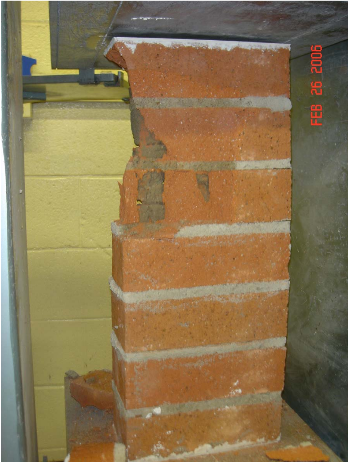
Figure 3.39: Prism with Approximate h/t Ratio of Five Built with Brick “C” and Type N Mortar Exhibiting Signs of Vertical Splitting and Face-Shell Separation Modes of Failure.
