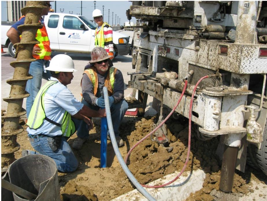
Figure 6.19 Water was filled into the casing to avoid floating due to buoyancy
