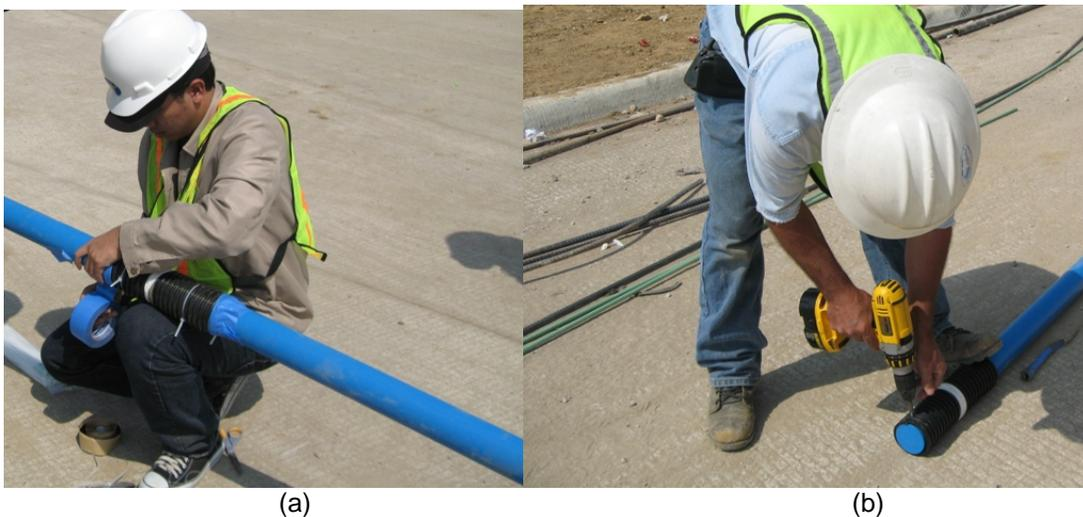
Figure 6.24 A corrugated pipe was attached on the casing with (a) mastic tape and (b) rivet
