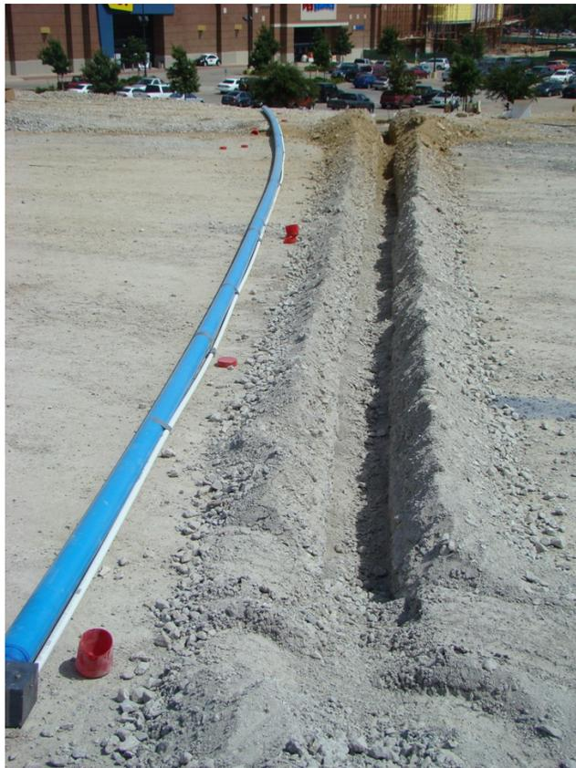
Figure 6.21 A trench was excavated at the selected location.
