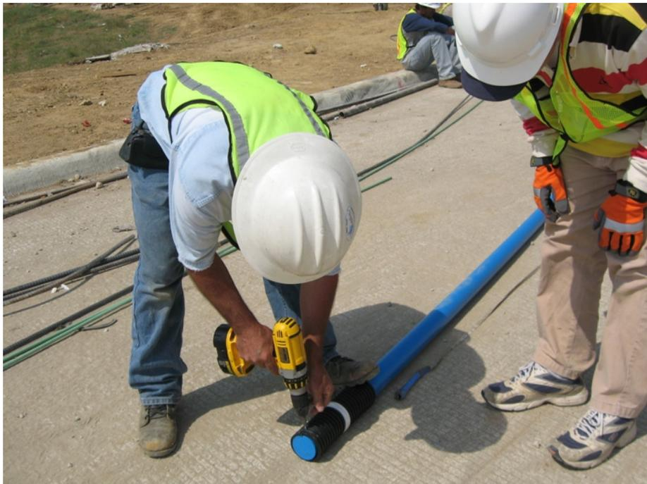
Figure 6.15 A bottom of the casing was plugged with a bottom cap
