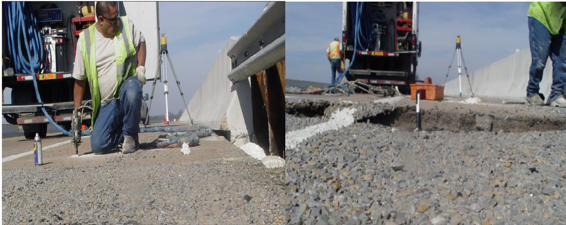
Figure 2.67 Position of approach slab during and after the Urethane injection process
