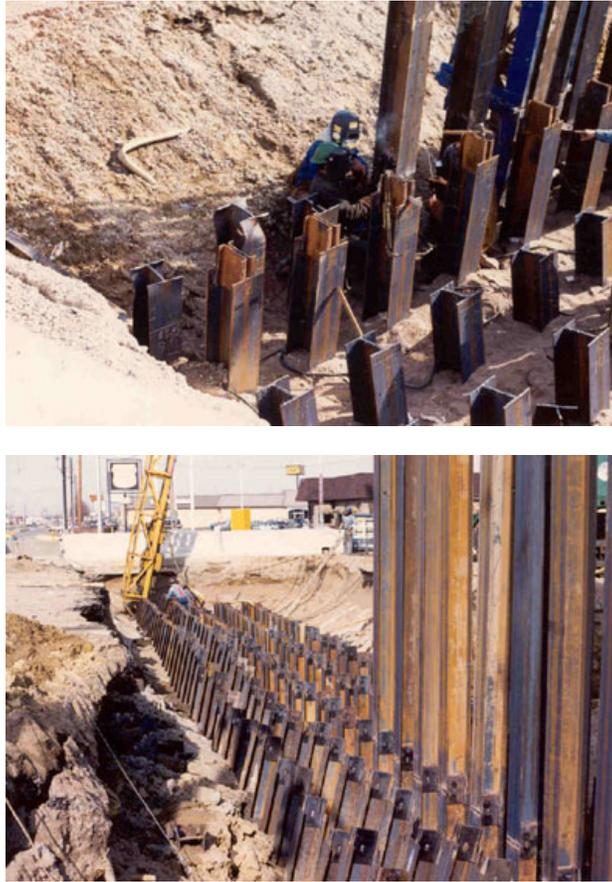
Figure 2.43 Example of Bridge Foundation using Steel H-Piles
