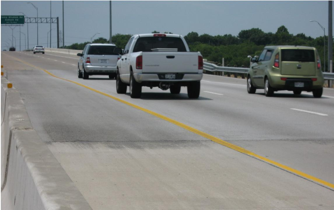
Figure 7.28 Bridge approach in the control embankment was overlaid by Asphalt to mitigate the bump
