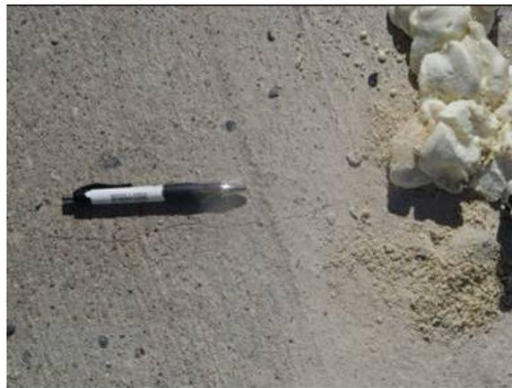
Figure 2.68 Hairline crack observed on the approach slab during the urethane injection
