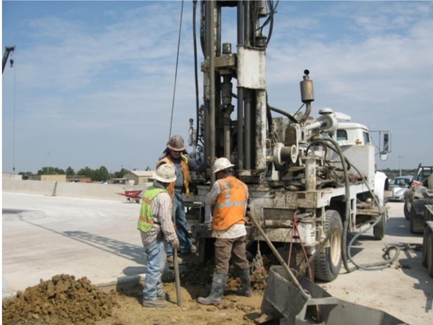
Figure 6.14 A selected location was bored to install the inclinometer casing
