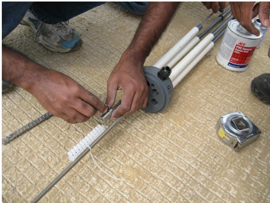
Figure 6.32 The VW sensor adapters were screwed into the reference head
