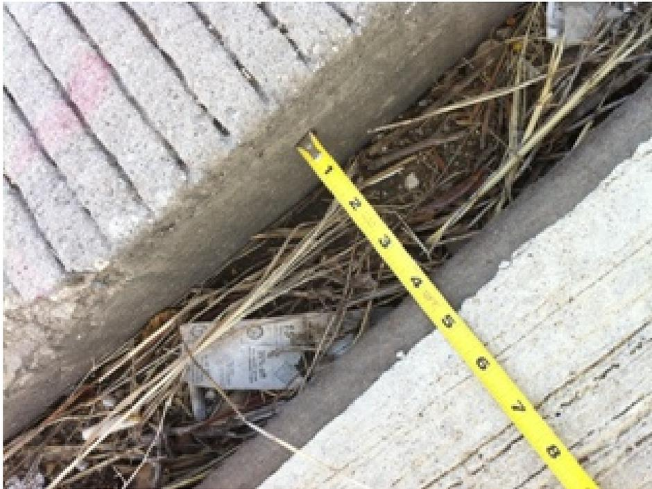
Figure 7.24 Lateral movement of the platform casing V4
