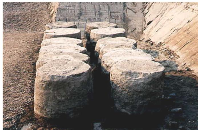
Figure 2.28 Deep Soil Mixing (DSM) Operation and Extruded DSM Columns
