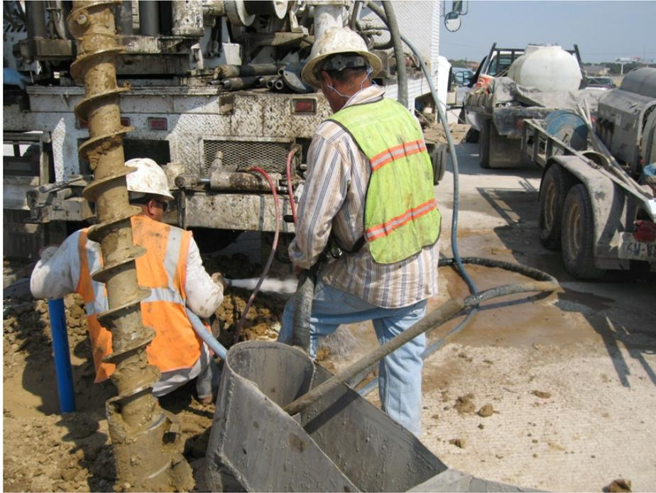
Figure 6.18 The gap between casings and bore was filled with grout mixing
