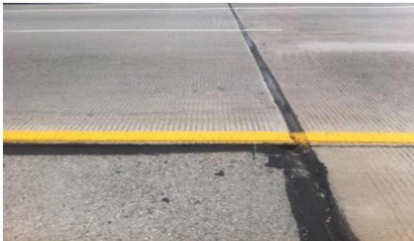
Figure 5.5 Horizontal movements on ECS section
