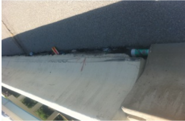
Figure 5.10 Vertical displacement at SH 360 -Control Section
