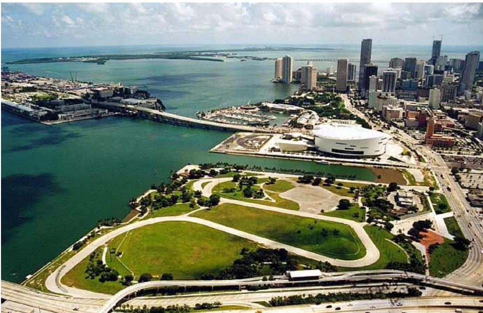
Figure 3.4 Port of Miami Tunnel Project (Image taken from http://www.portofmiamitunnel.com/images.html )
