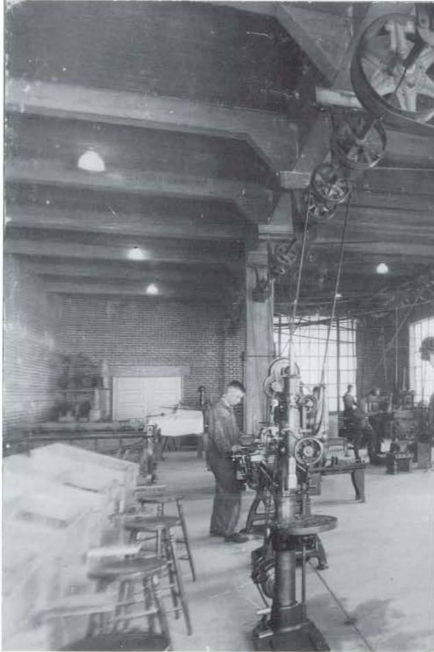
4.10 Although the college had a lower enrollment due to U.S. involvement in World War I, trades courses, such as auto mechanics, electric shop, welding, woodworking, and carpentry, helped to increase male enrollment by the early 1920s.
