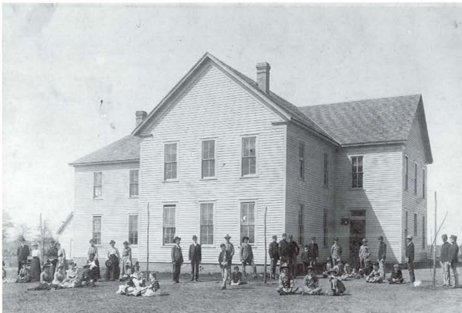
2.2 After moving from Hillsboro to Arlington, James M. Carlisle erected this wood-frame structure, the second building on campus. The different age groups and genders reveal the diversity of the 1902-1903 student body.
