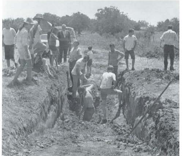
8.16 While the buried elephants have become a campus mystery, these photographs reveal the excavation as nothing more than a geology project.
