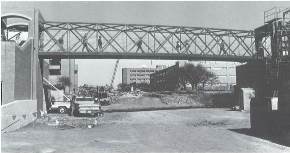
7.32 Noted as a hazard as early as the mid-1960s, the Cooper Street crossing problem was finally solved in 1990, when the street was partially depressed and three walkways were constructed over it.
