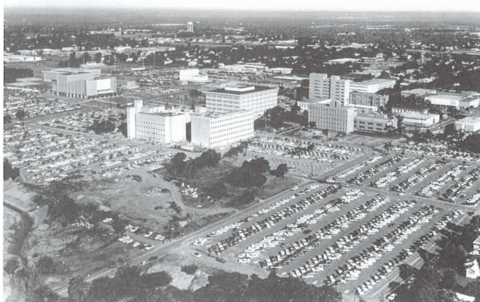
6.14 The characterization of ASC as “an island of enlightenment among a sea of parking lots” accurately describes this aerial view of the college in the late 1960s.
