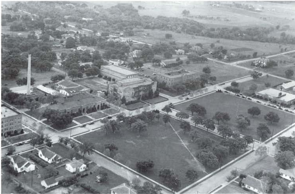
5.2 By the late 1940s, the North Texas Agricultural College campus had assumed a familiar look. Centered on west Second Street, the main campus occupied eight city blocks.
