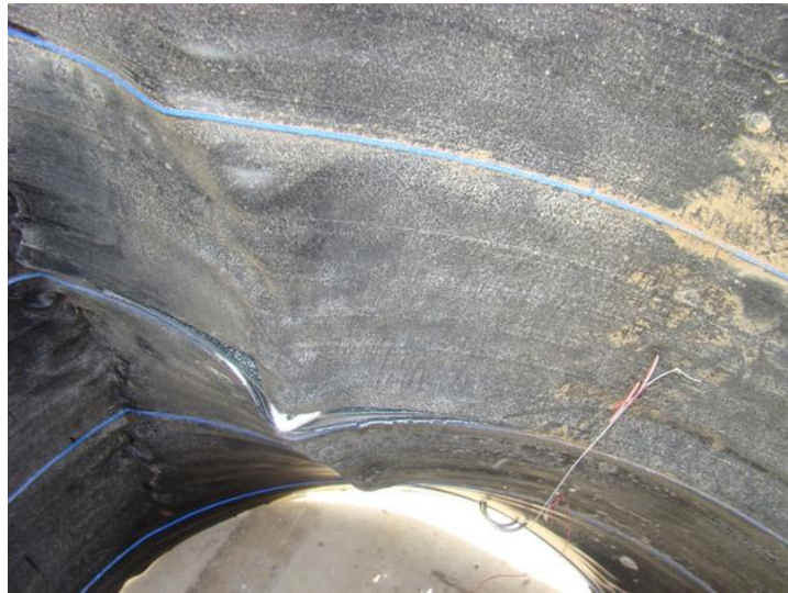
Figure 3.40 SR-HDPE 48 in. (122 cm) Pipe from Inside after Testing.
