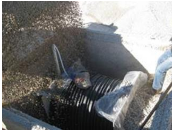
Figure 2.31 Filing the Box with \frac{3}{4} in. Gravel
