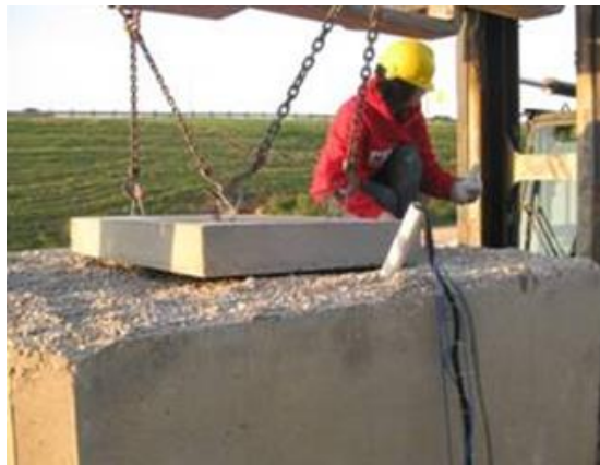
Figure 2.34 Slab Position on Top of the Box
