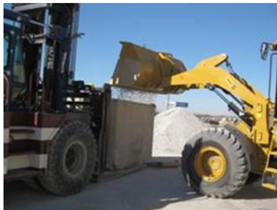
Figure 2.32 Filing the Pipe up to Crown Level
