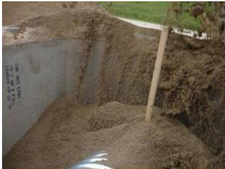
Figure 2.21 Filling the Box at 6 increments
