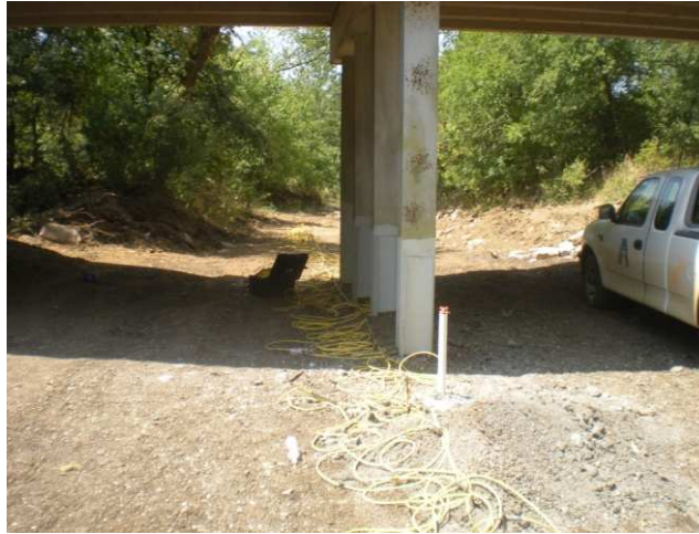
Figure 3.16 Resistivity Set up for Mountain Creek on FM 2738
