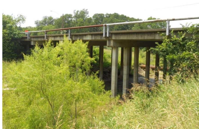
Figure 3.4 Site Picture of Bridge sites (02-220-0008-06-052)
