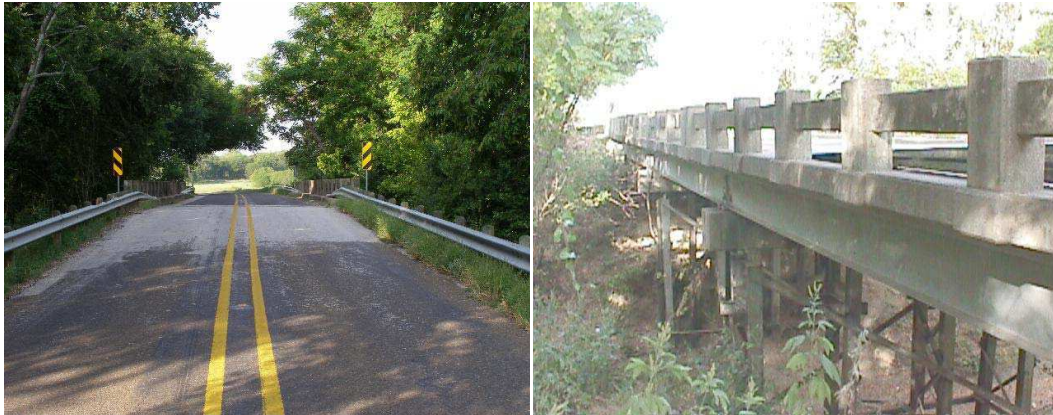
Figure 3.2 Site Photos of Bridge at FM916 over Chambers Creek
