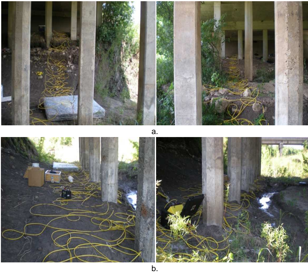
Figure 3.14 RI test at bridge on Division Street, Arlington, a. 2D resistivity field set up, b. 3D resistivity field set up.
