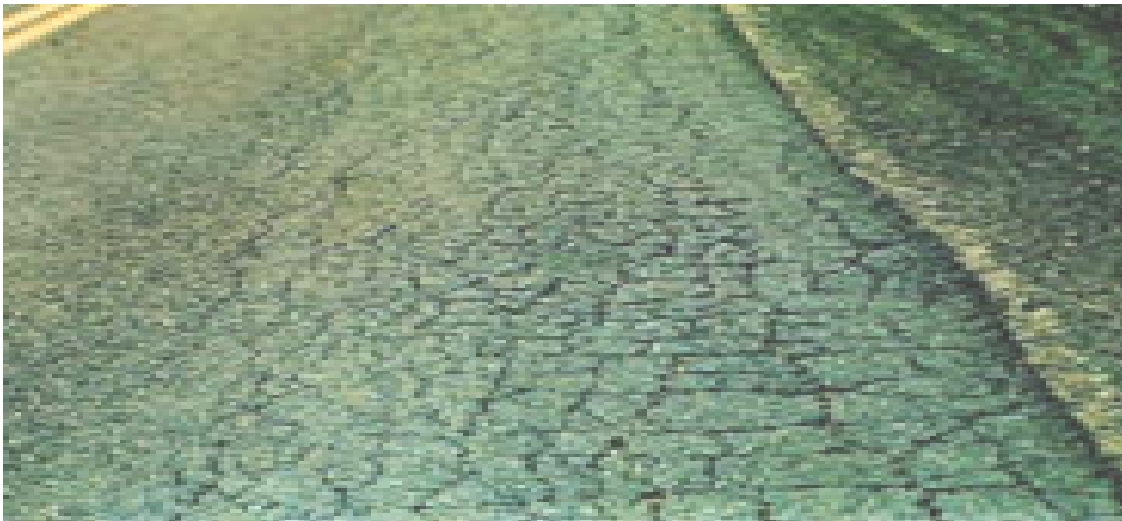
Figure 2.2: Alligator Cracking
