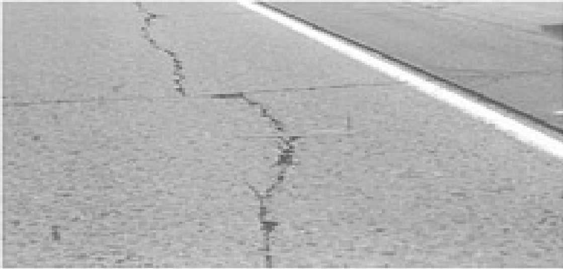
Figure 2.4: Longitudinal Cracking
