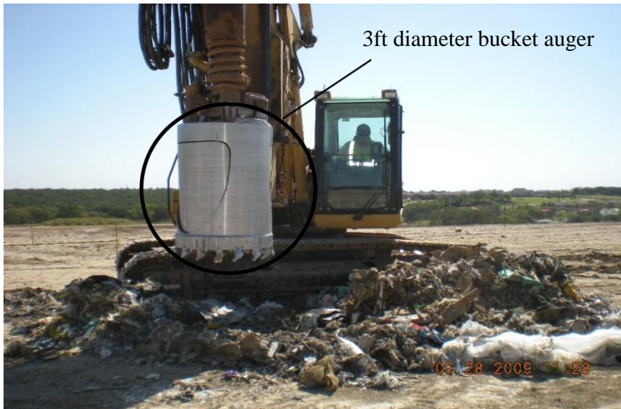
Figure 3.4 Borehole Samples Collection Using 3ft Diameter Bucket Auger
