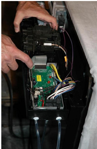
Figure 2.3. PCB located inside door panel assembly - Note injection ports tubes located at bottom of picture (courtesy: St. Joseph Technology Center).
