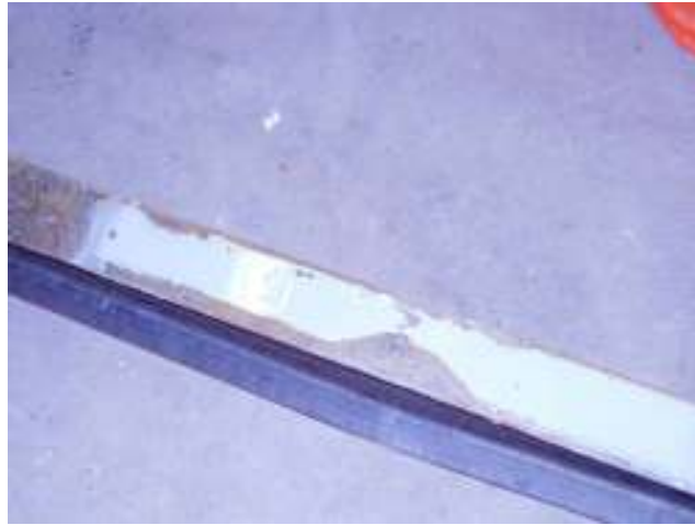
Figure 3.4: Proper de-lamination of CFRP
