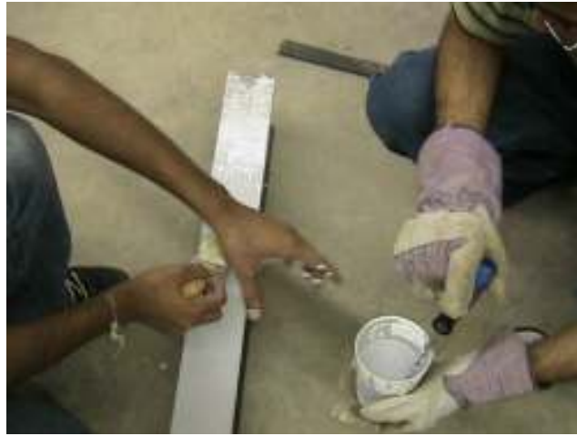
Figure 2.7: Applying epoxy to CFRP laminate
