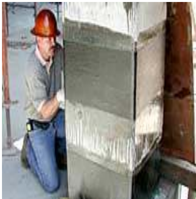
Figure 1.3: Removal of air voids during hand lay-up sheet CFRP [18]
