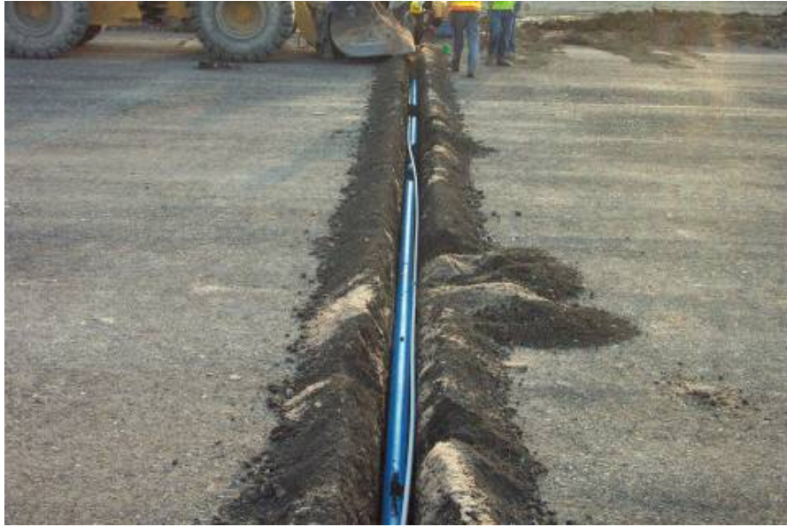
Figure 5.4 Horizontal Inclinometer Installation
