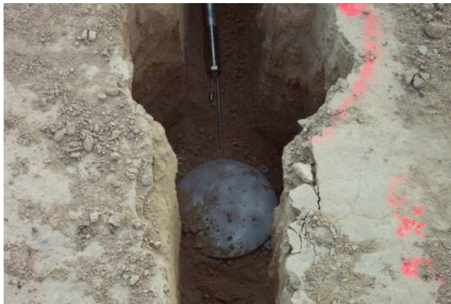
Figure 5.9 Installation of Pressure Cells
