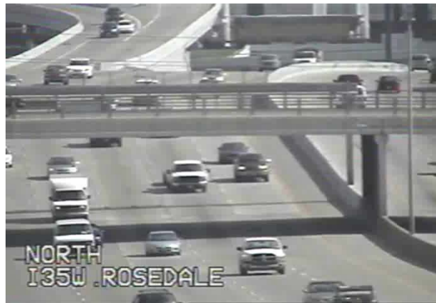
Figure 1.3 Traffic video snapshot at low vibration frequency of the pole.
