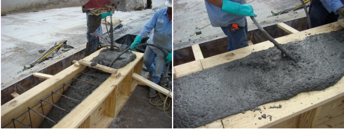
Figure 3.8 Typical photos of casting concrete
