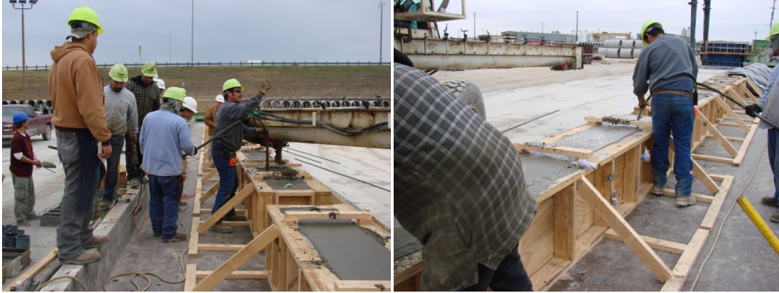
Figure 3.15 Typical photos of casting – the second phase study
