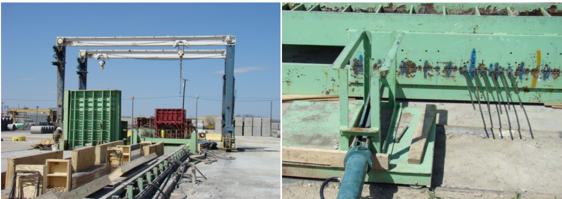
Figure 3.7 Prestressing bed and jacking in Hanson Pipe & Precast Plant
