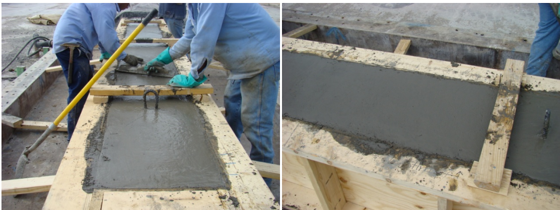
Figure 3.10 Finishing surface
