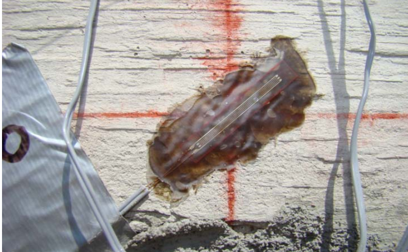
Figure 3.20 Example of concrete surface strain gage
