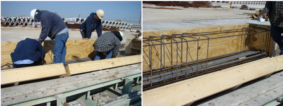
Figure 3.6 Typical photos of reinforcement caging
