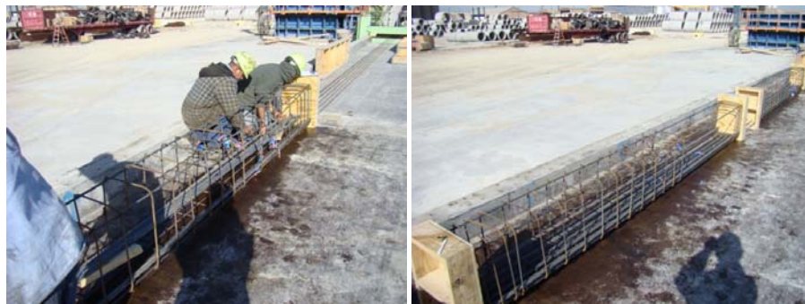
Figure 3.14 Typical photos of reinforcement caging – the second phase study
