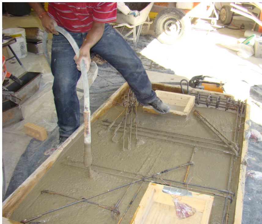
Figure 4.7 Consolidation of concrete by vibrator
