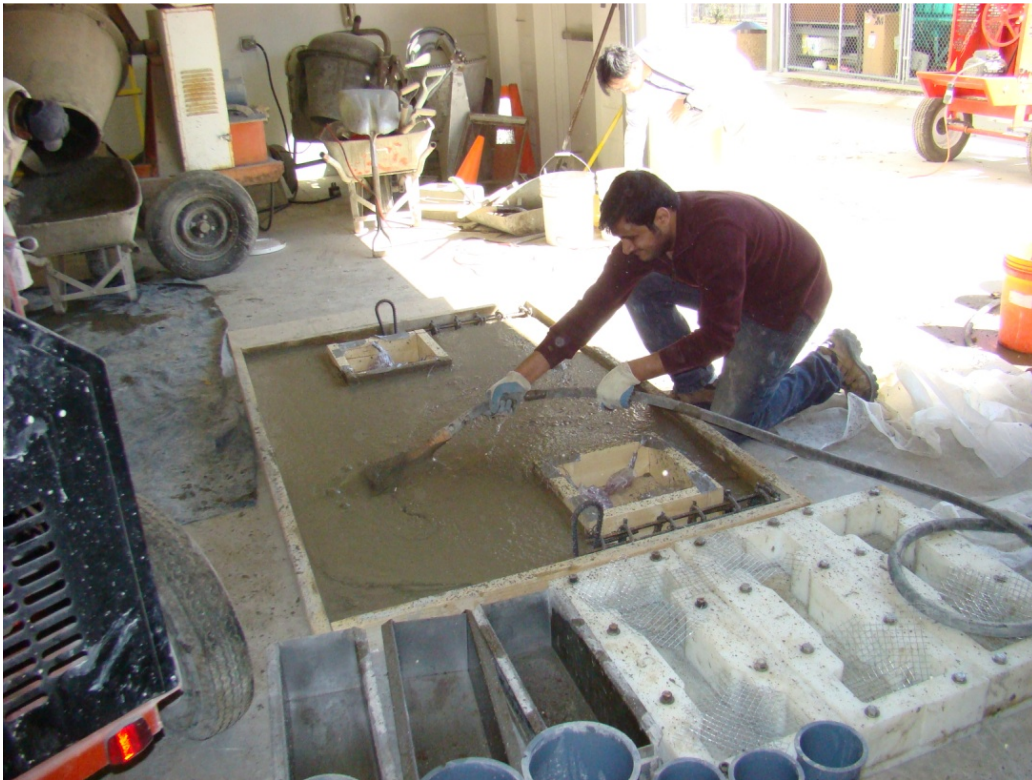
Figure 4.31 SFRC #1 test specimen during placing and consolidation of plastic concrete
