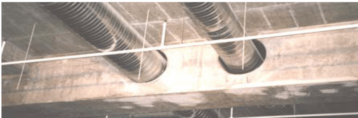
Figure 1.2 Concrete beam with large circular openings (Amiri, 2011)
