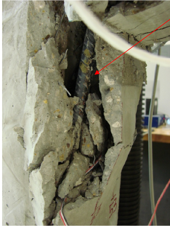
Figure 4.38 Observed debonding of rebar in SFRC #1 specimen
