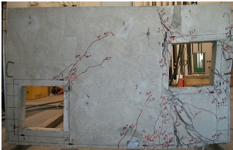
Figure 5.10 Non linear finite element analysis for SFRC#3: Cracking pattern at ultimate load of 60 kips (267 kN)
