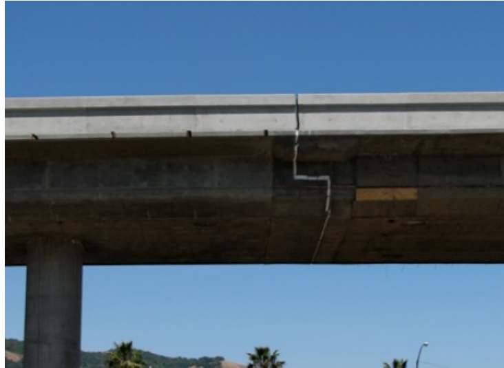
Figure 2.5 In-span hinges in RC box-girder bridges (Interstate 580 connector, San Rafael)
