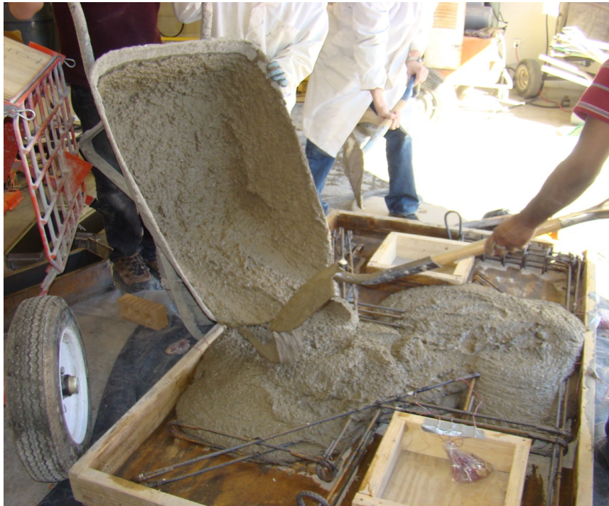
Figure 4.6 Concrete pouring for RC specimen
