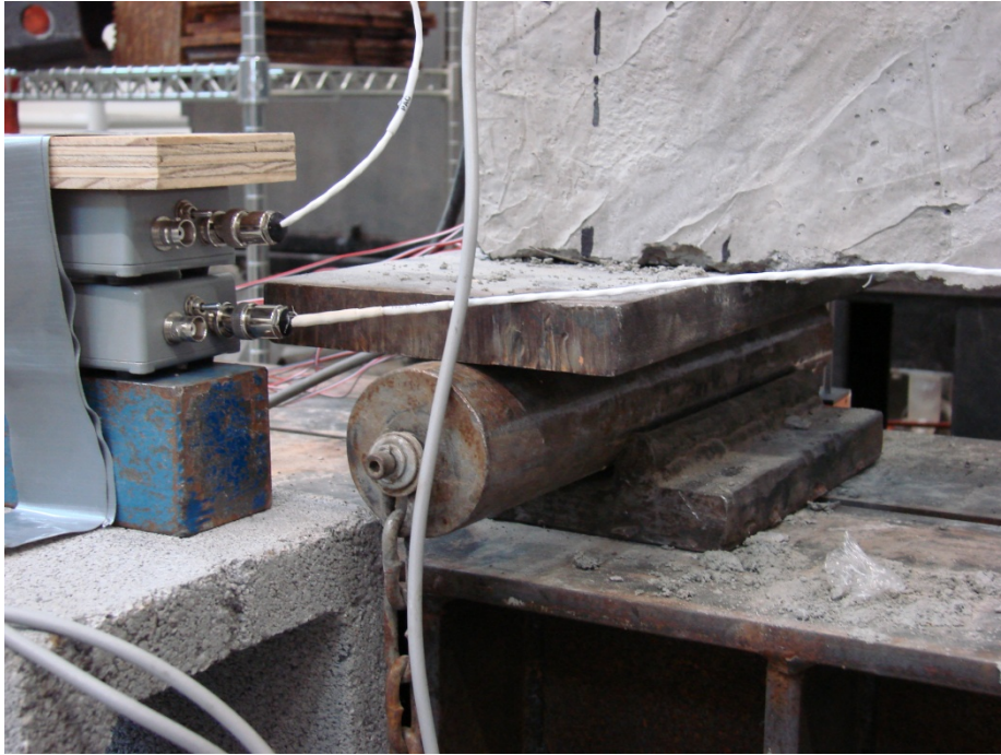
Figure 4.33 Pre-Crushing of concrete near the support of SFRC#1 specimen
