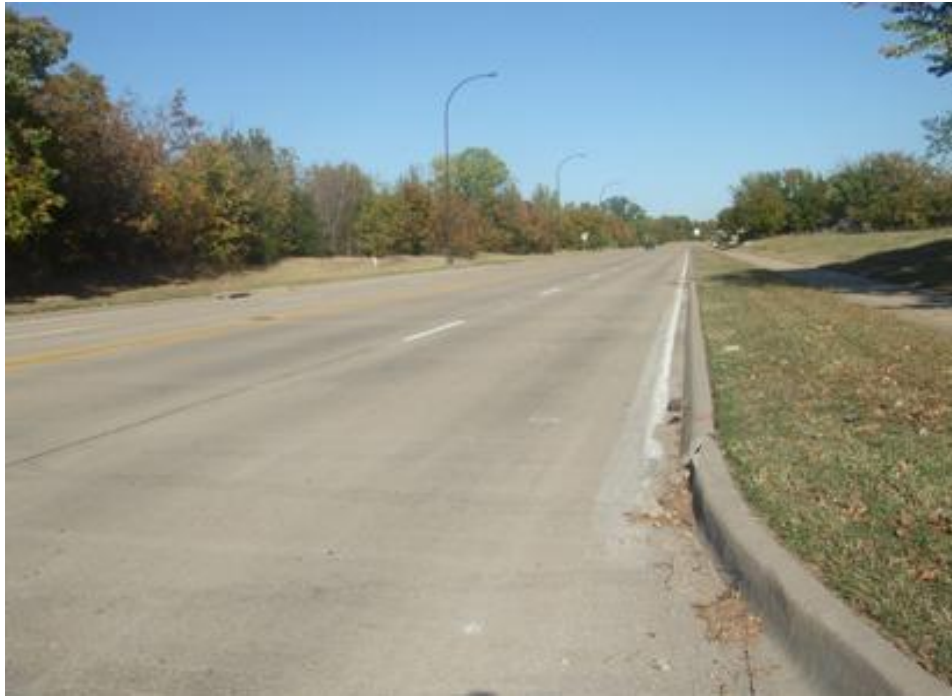
Figure 3.1 Abram Street (PCC).
